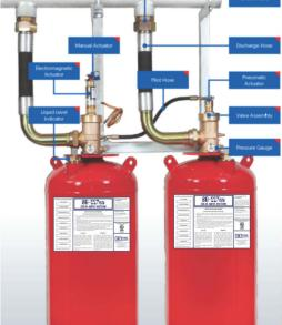
The cylinders are available with both mild steel welded type of TPED 2010/35/EU Standard and Chromium Molybdenum Alloy Steel Seamless type of ISO 9809-1 Standard.
